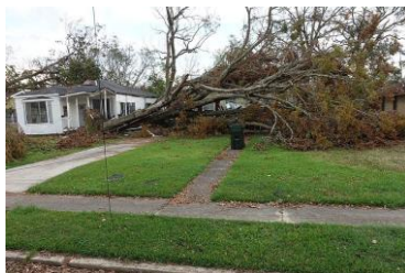
Massive storm damage in Lake Charles, LA
